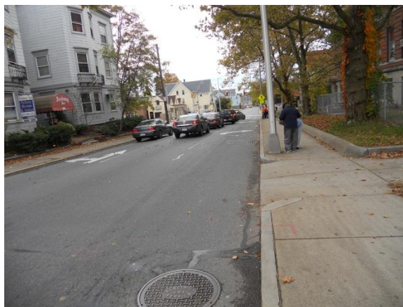
Lack of lane control signage on Warren Avenue approach
