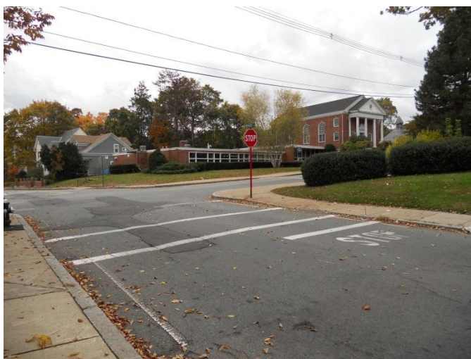
Dual Stop lines and set back Stop signs on Newbury Street southbound approach
