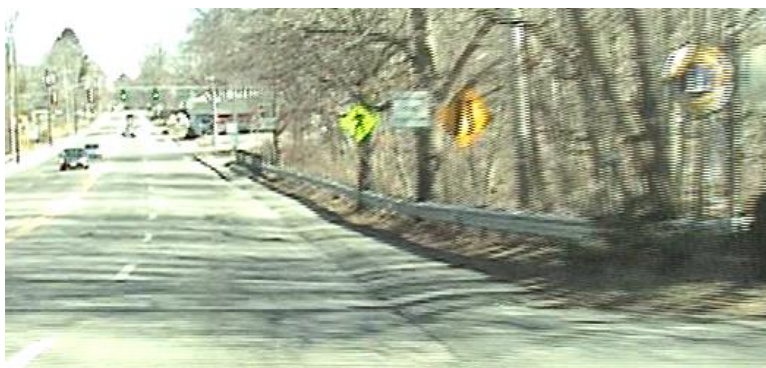
Sign Clutter approaching Whitman Street
