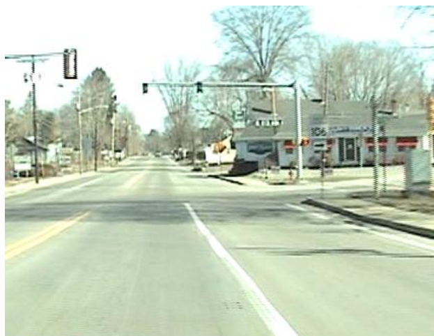
Mast Arm (April 2014)
