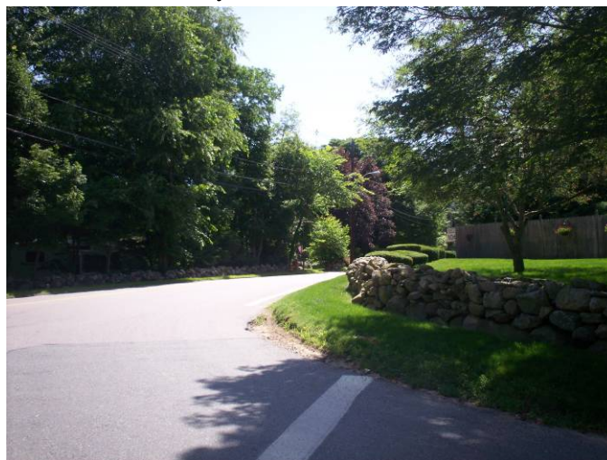
Sight Obstructions looking east on Foundry Street from Prospect Street
