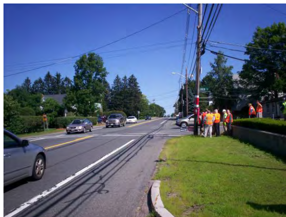
Existing Crosswalk at Union Street
