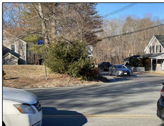
Sight line blocked on the Depot Street approach by a berm and vegetation looking north toward Turnpike Street.
