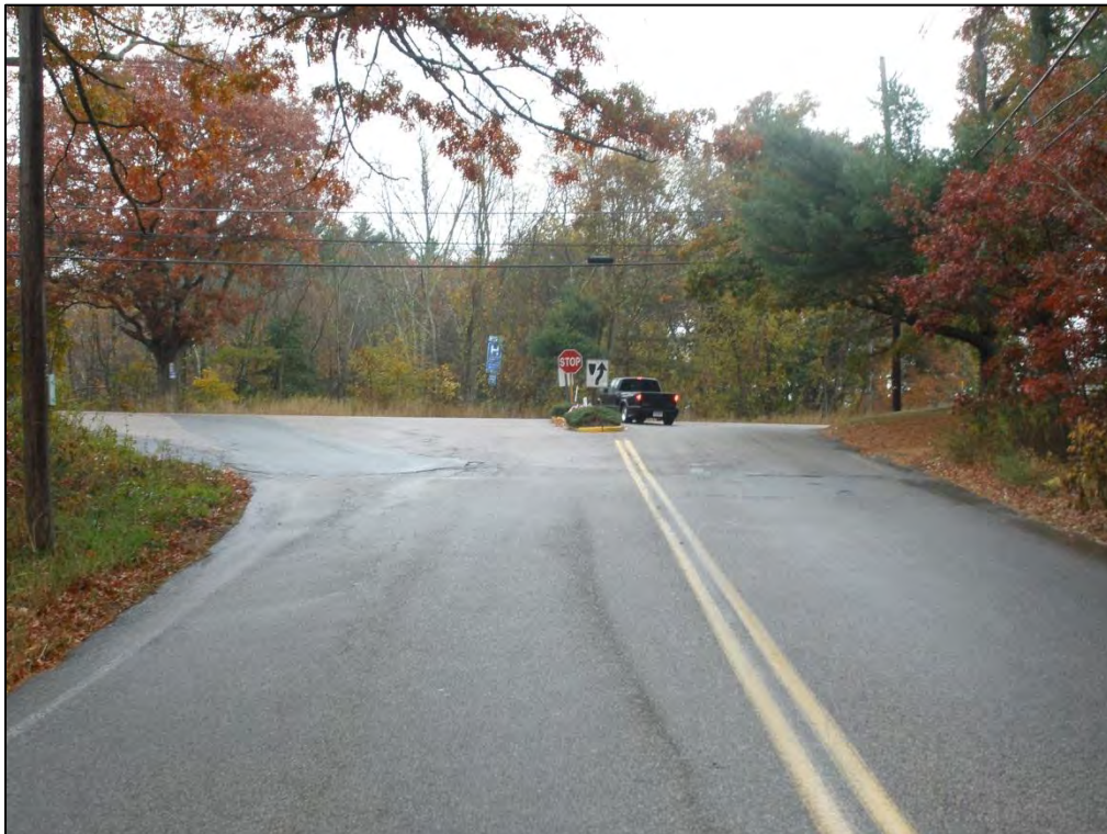
Elm Street approach to the Elm Street/Main Street (Route 27) intersection showing ascending grade and island for channeling traffic
