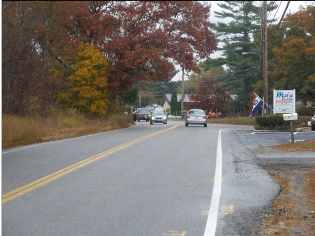
Main Street (Route 27) southbound approach to the Elm Street/Main Street (Route 27) intersection showing wide open curb cut to diner parking lot
