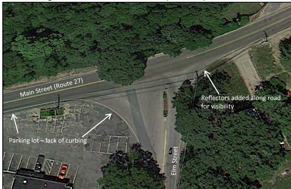
Figure 3 Elm Street/Main Street (Route 27) Intersection
