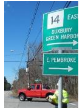
Bent sign corner
