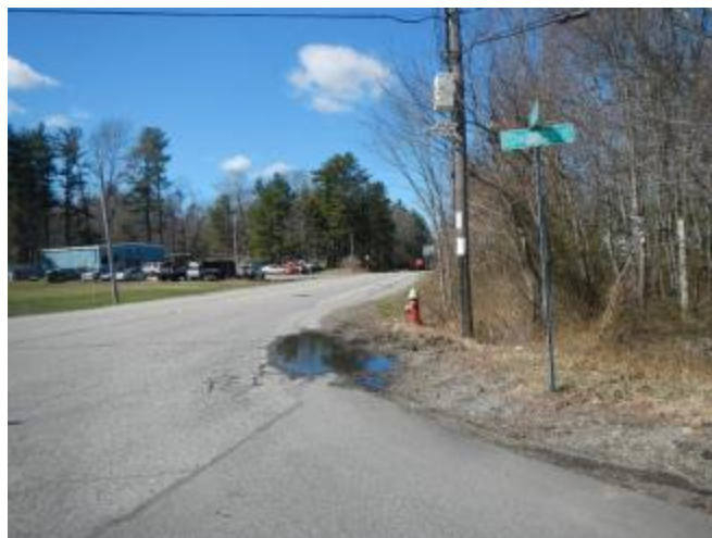
Vegetation growth on northeast corner
