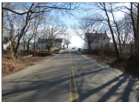
Nelson Street eastbound traffic sight distance is obscured by the house on the inside of the curve.
