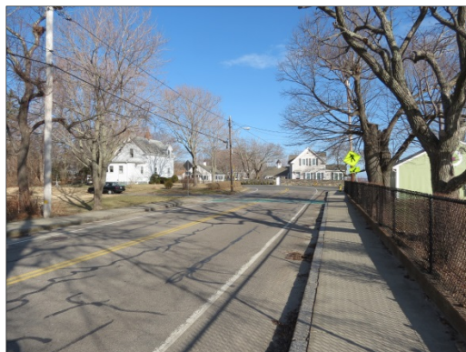
Water Street northbound traffic sight distance is obscured by roadside vegetation and sharp curve.
