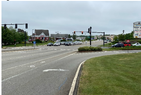
Image 1: Pedestrian crossing on high-speed free right turn lane increases hazard for pedestrians.
