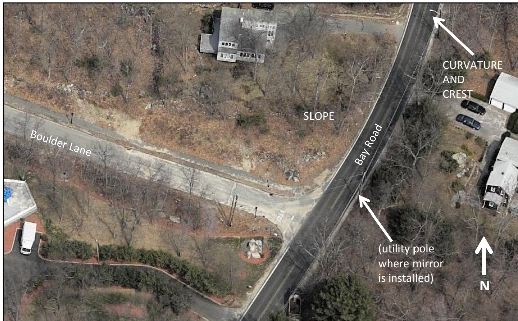
Bay Road/Boulder Lane intersection showing curve and grade crest on the southbound approach and slope with trees on the northwest side
