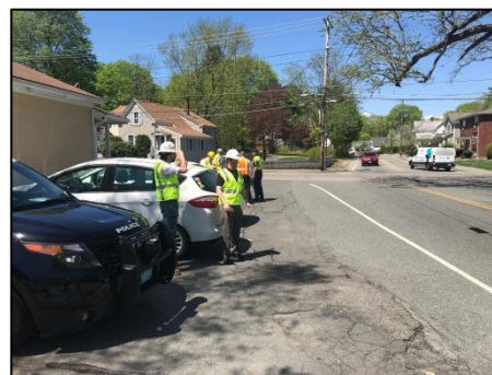
Lack of curbing on the south side of Lincoln Street to contain vehicles in the convenience store parking spaces.
