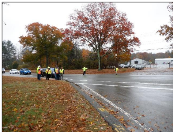
Vehicles turning right from Park Street northbound to Turnpike Street take the turn at high speeds due to the wide turning radii.
