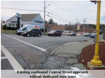
increasing the potential for crashes. The audit team stated that there are no pavement markings or signage along either Central Street approach indicating lane designations and they also noted that the left turn only lane utilization sign was missing from the mast arm for the northbound approach on Washington Street.
