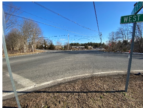
Image 1: The wide footprint of the intersection combined with set back stop bars creates a large distance between vehicles.
