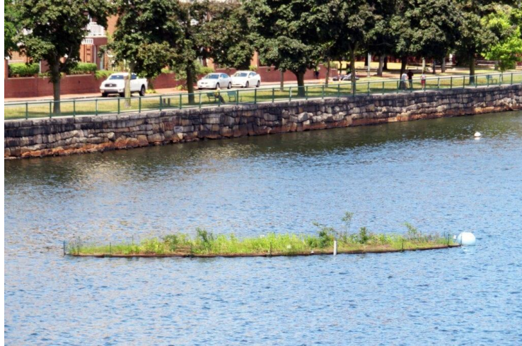
Charles River Floating Wetlands - improve water quality, control toxic algal blooms, and improve fish habitat and health.
