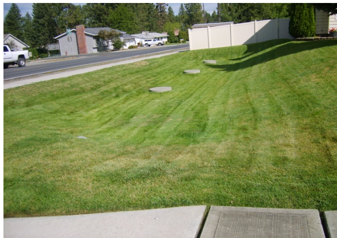
Figure 9: An example of a swale, with overflow storm drains
