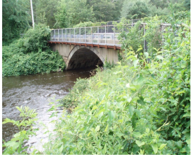
Figure 4: Bridge Street Bridge, Bridgewater, July 2011.
