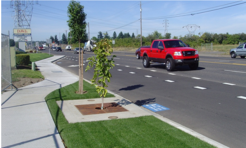
Figure 11: Tree box along a highway.
