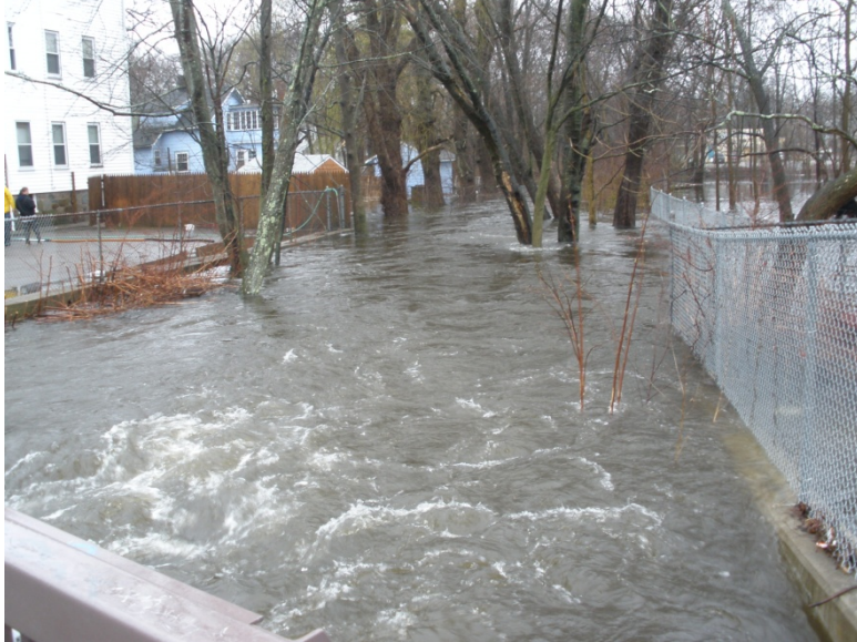
Figure 7: The Salisbury Brook overflowing near Pleasant Street (Route 27) in Brockton, March 2010.
