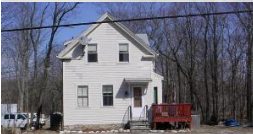
Above: 175 Turnpike Street, built 1900
