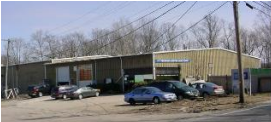
Above: 199 Turnpike Street, built 1978
