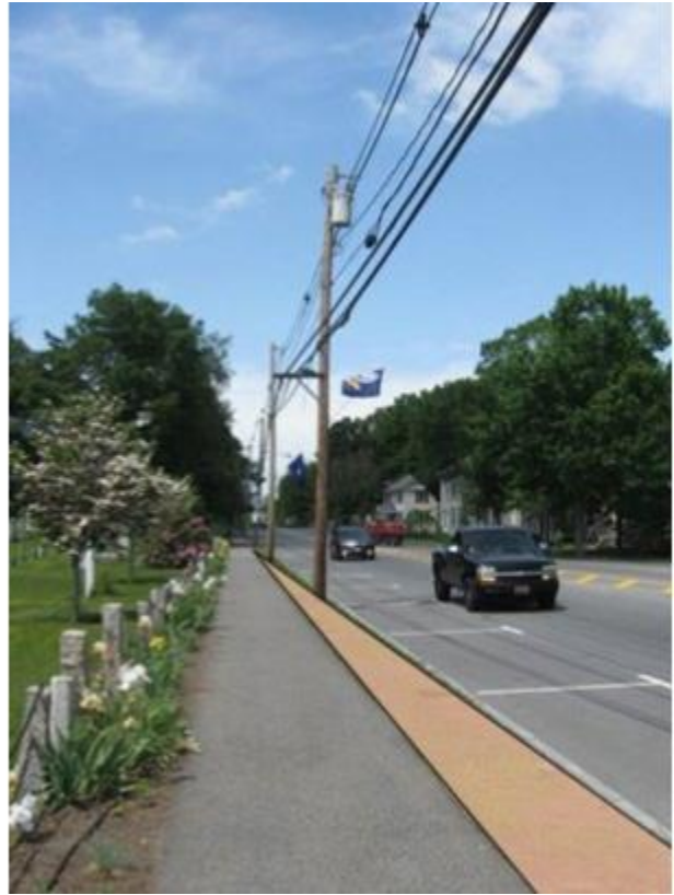
Consistent edge banding in brick or other materials may be preferable along curb edges where there is parallel parking and where the landscape is subject to winter time damage associated with salting and plowing.
