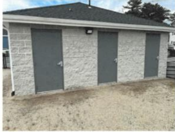
Park Side Restroom Entrances
