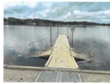
Close up of Swim Access and dock
