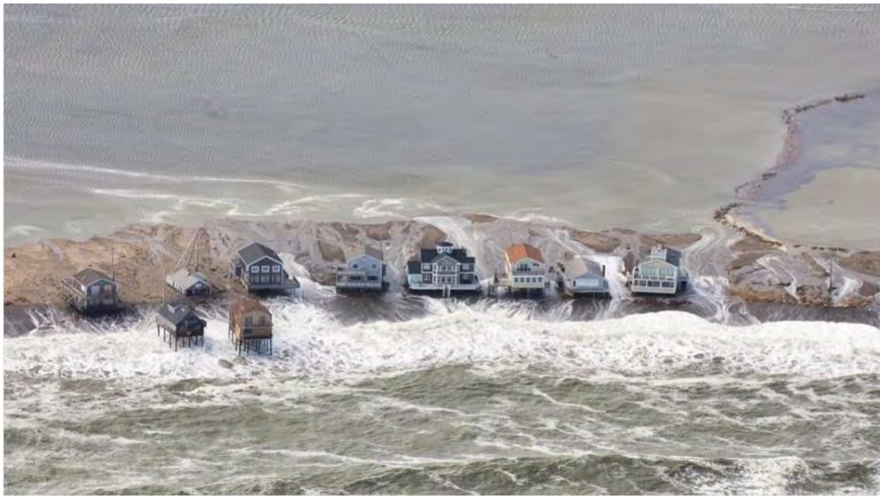
Figure 72: March 2018 Storm Surge
