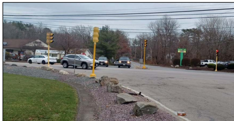
This photo shows the eastbound approach is not lined up with the receiving lane. In addition, the approach lane is wide enough for two vehicles to stack side by side on the approach, but the intersection is lacking proper pavement markings indicating lane use.
