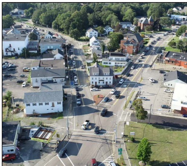
Southbound queues on Central Street during the PM peak hour extend from the Spring Street/Central Street/Maple Avenue intersection through the Central Street/North Central Street/Union Street intersection.
