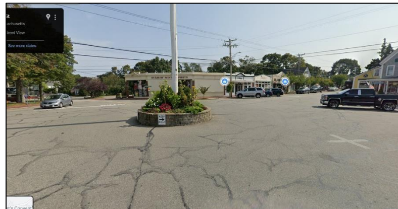
The only control indicating traffic flow direction in the circle is a “Keep Right” sign on the low wall around the flagpole in the center.
