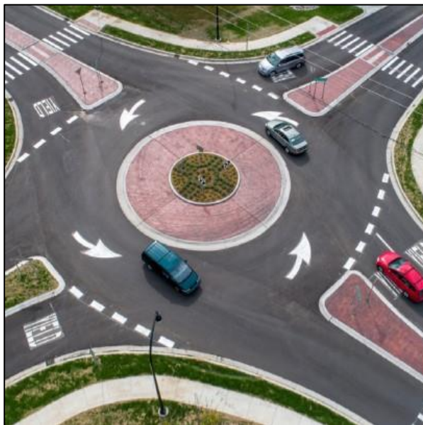
An illustration of a mini roundabout with mountable apron and mountable splitter islands on approaches. In addition, crosswalks and pedestrian refuge islands are included for safe pedestrian crossings.
