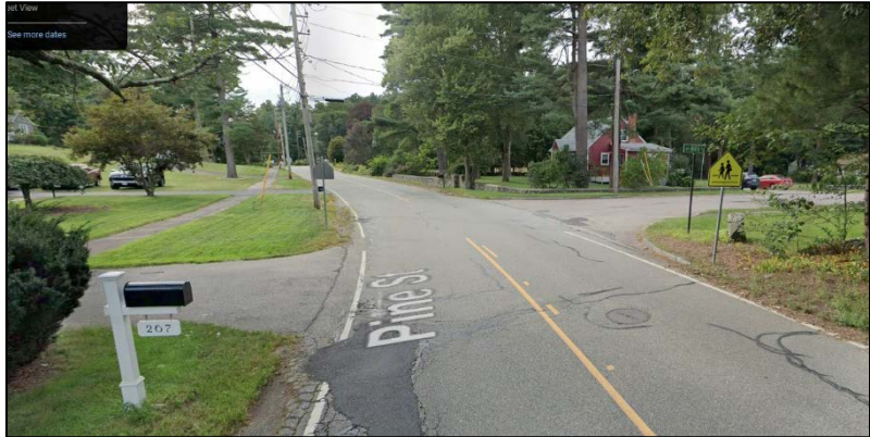
Photo above shows the lack of a crosswalk across Pine Street at Ruth Road at the pedestrian crossing sign as well as the faded DYCL.
