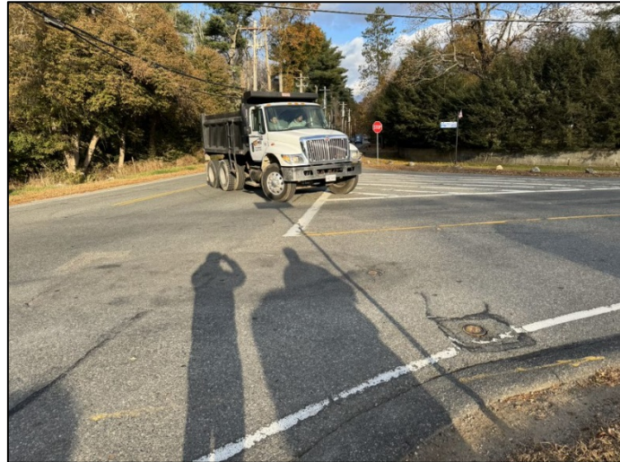
Photo above shows a left turn from Plain Street westbound to West Street southbound encroaching on the painted island. Also shown is the stop sign at the end on the painted island on the West Street northbound approach.
