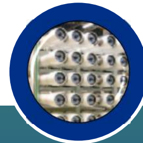
Reverse Osmosis Membranes
