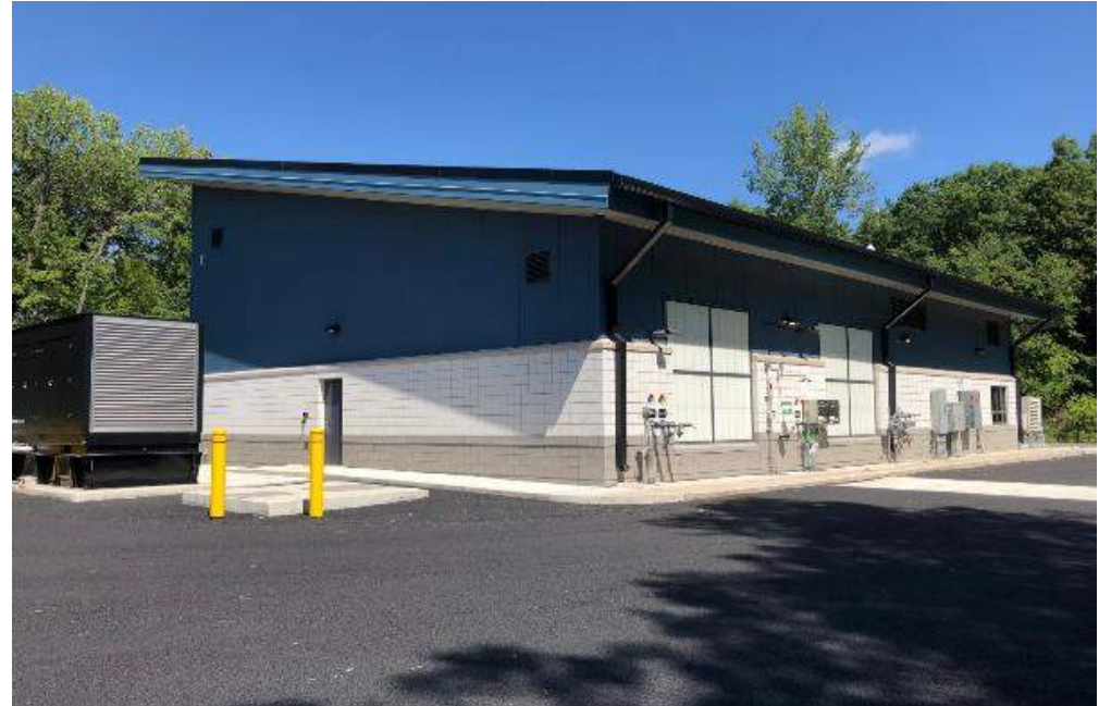
Owen District Road Water Treatment Plant Westfield, Massachusetts
