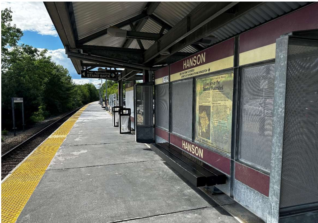
Figure 19: Image of Commuter Rail in Hanson
