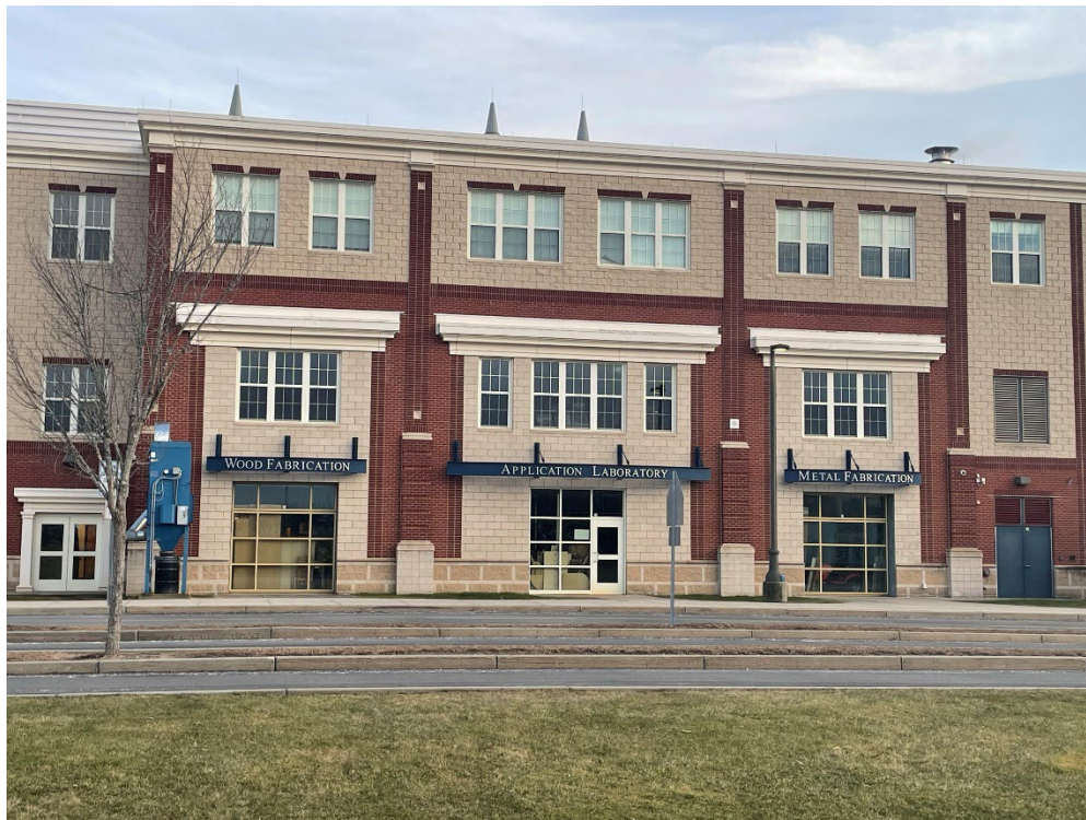
Figure 23: East Bridgewater High School
