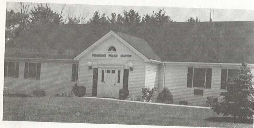
Pembroke Police Station
