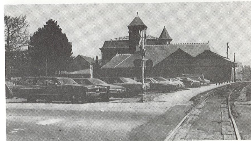
Stoughton Train Station
