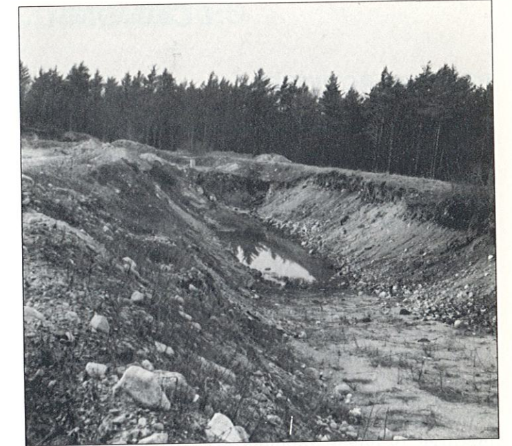
Typical Lagoon Under Construction
