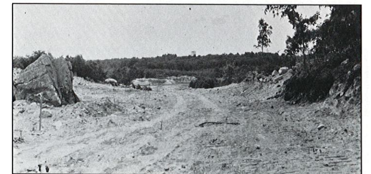
Avon Industrial Park-West Roadway
