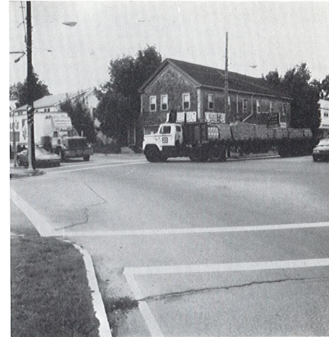
Route 106/28 intersection in West Bridgewater looking westward
