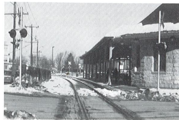
Renovated Stoughton Commuter Rail Station
