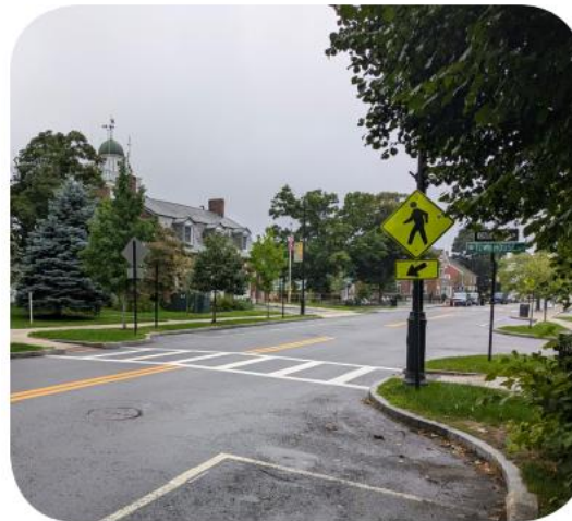
Curb extensions shorten the pedestrian crossing distance and enhance visibility.
